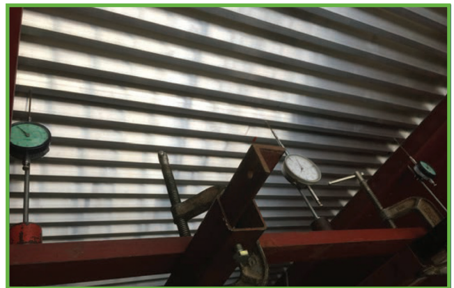
Internal View of Horizontal line load test
